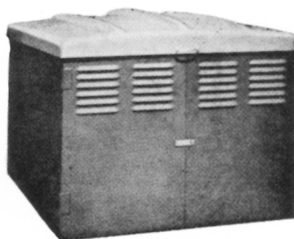
FIGURE A.3.3.16(b) Steel Hose House of Compact Dimensions for Installation over Private Hydrant. House is shown closed; top lifts up, and doors on front side open for complete accessibility.
